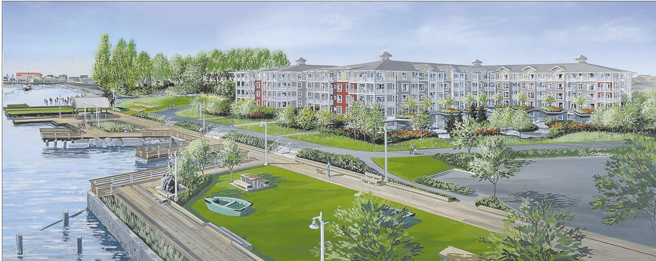
The Copper Sky project at Imperial landing in the Steveston Village area of Richmond is a 91-unit condominium development by the Omni Group due for completion in June.
